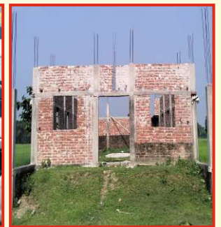
Parul Church Construction in Progress
